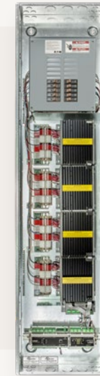
GLCAEN-MLO SpaceBuilder System SpaceBuilder Main Lug Panel
