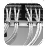
**CAUTION:** Do not overtighten the cable ties, as this may deform the cable jackets and may lead to decreased transmission performance.
