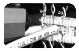
**NOTE**: Ensure that the punch tool is in perpendicular alignment with the conductor during termination. Do not attempt to terminate the conductors at an angle.
