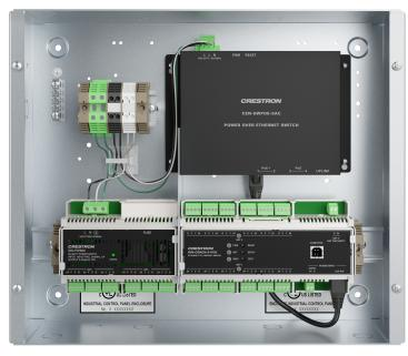
The Crestron® ZUML-CENCN-SWPOE-5 is a preassembled lighting network expansion panel that expands Ethernet and Cresnet® network connectivity for a Crestron lighting system. It contains a DIN-CENCN-2-POE Ethernet to Cresnet Bridge, DIN-PWS60 60 Watt Cresnet Power Supply, and CEN-SWPOE-5AC 5-Port PoE Switch all mounted in a DIN-EN-2X18 wall mount enclosure.
